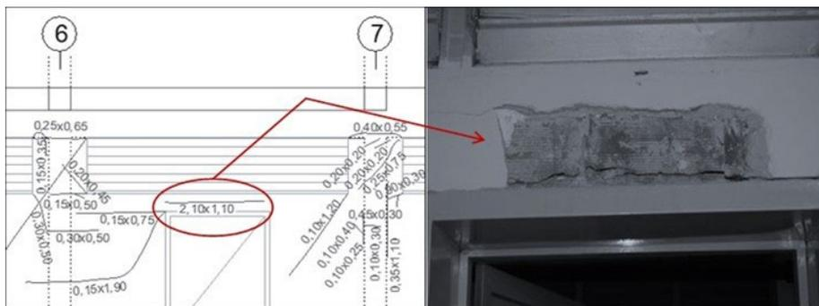
Figure 11. Example of the registration of cracks.
