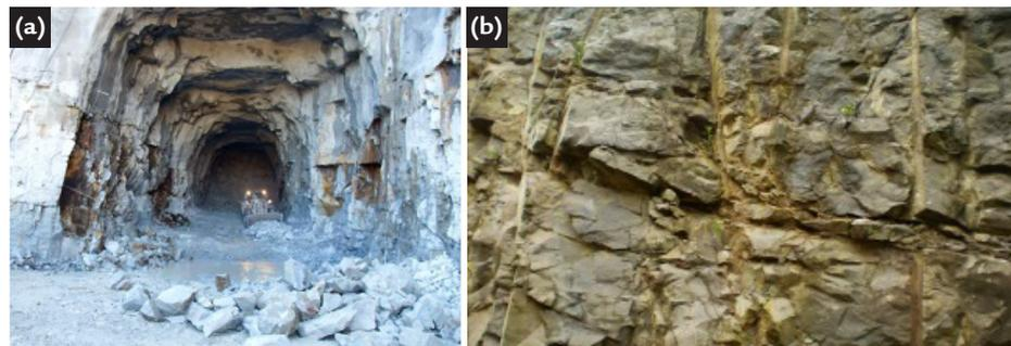
Figure 2 - (a) Overbreak generated by geological structures (discontinuities). (b) Sample of overbreak generated by deviations from controlled holes.
